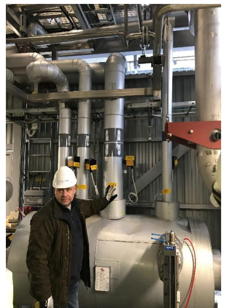
Krister Håkansson explain functions of the condensate tank
